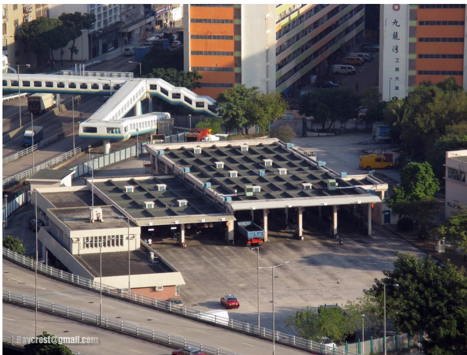
Figure 6-1 Vehicle Examination Centre – Kowloon Bay
