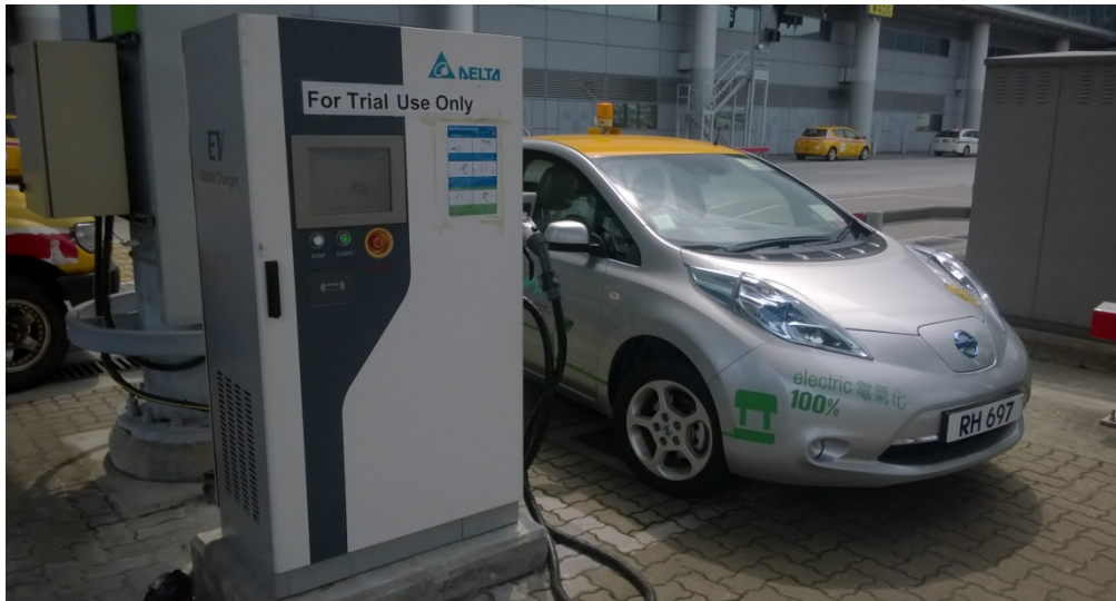
Figure 4-4 DC Quick charging EVSE
