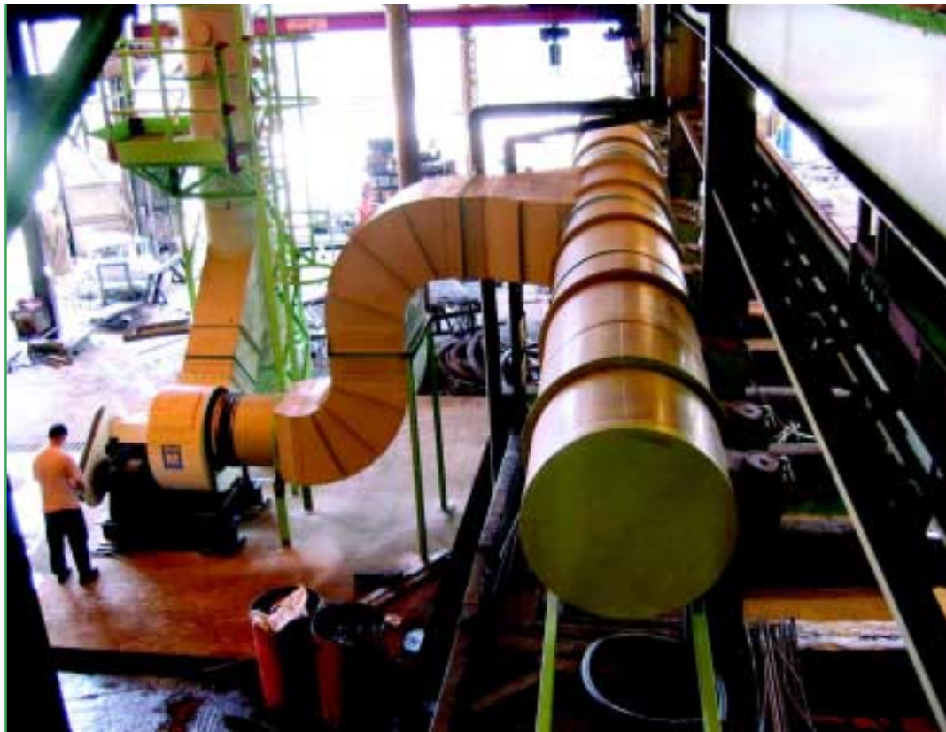
生產力局為本港一家熱浸鍍鋅廠設計及安裝廢氣處理設施。 An air pollution control facility designed and installed by HKPC for a hot-dip zinc galvanizing factory in Hong Kong.
