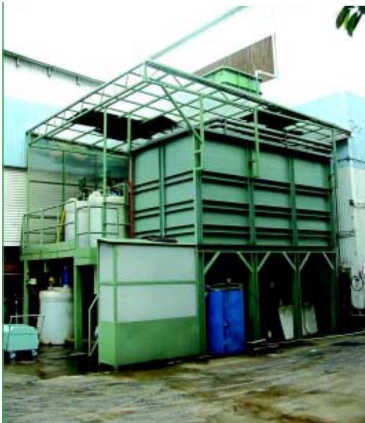
生產力局為一家位於大埔的鋁廠設立污水處理系統。 A wastewater treatment plant set up by HKPC for an aluminium work company in Tai Po.
